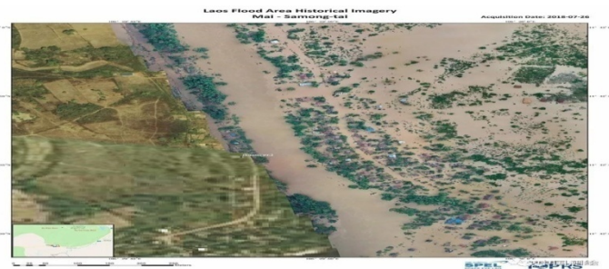
Dam failure in southern Laos
